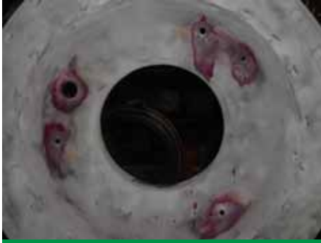
1 Cleaning/inspection incl MPI/dye check (pressure test)
